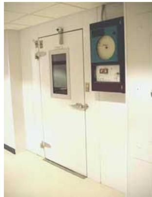
Air conditioned rooms
